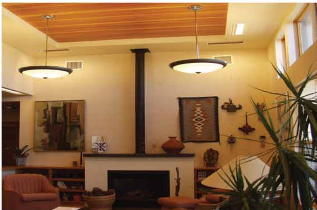
Daylight in this condominium has been balanced with ambient light from dimmable hanging fluorescent ceiling fixtures. These fixtures bounce light off the ceiling and provide light downward. This type of fixture is referred to as a direct/indirect fixture.
