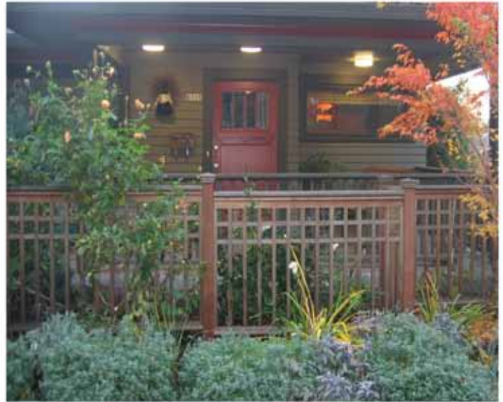
Ambient light is provided for this front porch by surface mounted porch ceiling fixtures with diffusing lenses. These fixtures provide light for the walkway, the house numbers and on the face of a visitor at the door, leaving no dark corners for an intruder to hide.
