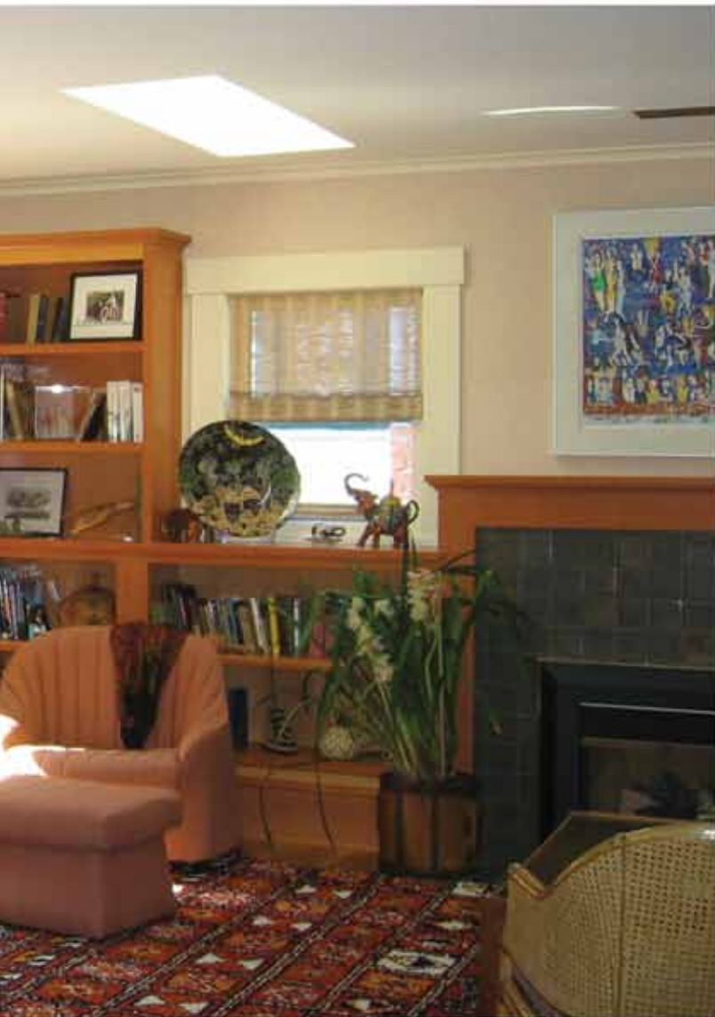
A skylight was added to the living room of this 1920's style bungalow to help balance the daylight coming from the windows and provide high light levels during the day.
