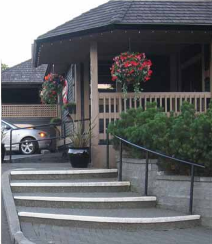
These steps are clearly marked with a white line, providing an excellent visual cue that will help to prevent falls. By providing edges with a contrasting strip, everyone can see better, especially at night.
