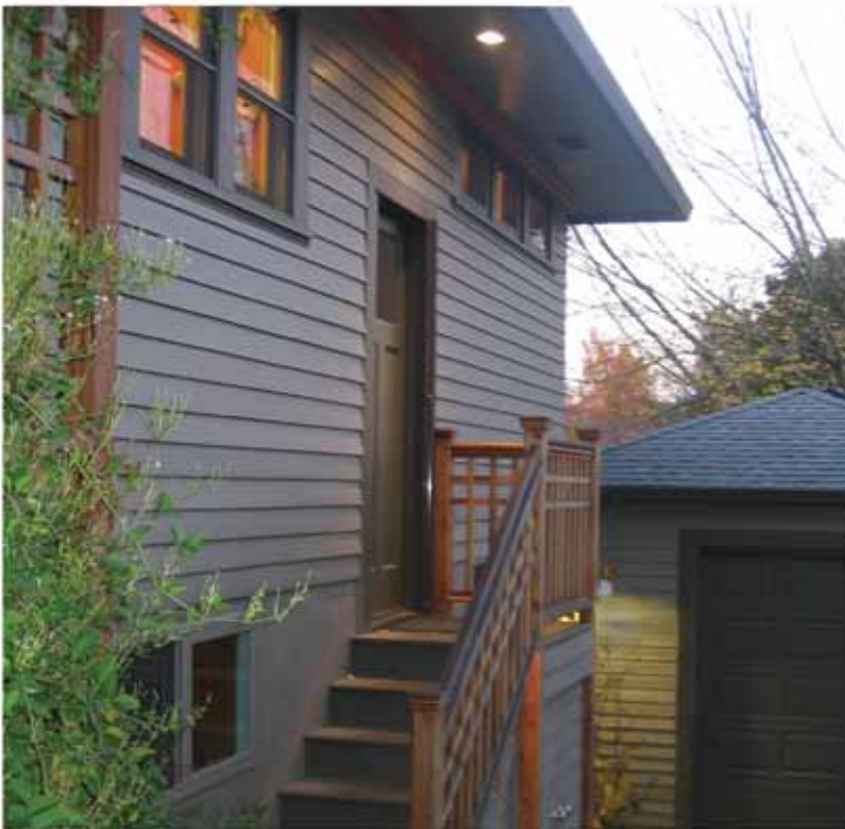
This back porch utilizes two light sources. The recessed downlight provides light onto the door and landing area. A rope-light mounted under the lower rail provides light on the stair tread, while concealing the light from the eyes. This is also an excellent way to provide lighting for interior stairs.
